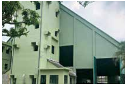
Igloo building after renovation
