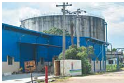
New warehouse in Lot 39C
